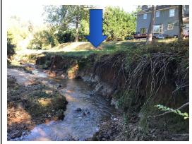
In this picture, the extreme erosion of the streambank has put the driveway of this house at-risk of damage or failure. Continued erosion could result in permanent damages to the road/ property. (ReWa)
